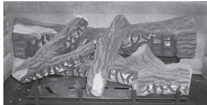
Logs D)02-46 and E)02-47 in position.
